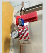
Lockout/tagout (LOTO) equipment consists of tags, locks, hasps, chains, and other hardware used to prevent the operation of equipment being serviced or maintained. Lockout devices must be used whenever possible, to ensure a positive means of energy control, by holding equipment in a SAFE or OFF position. Tags should be used in conjunction with lockout devices to warn against operation.
